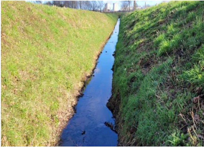
Photograph 7: Typical on-Site ditch (D2).
